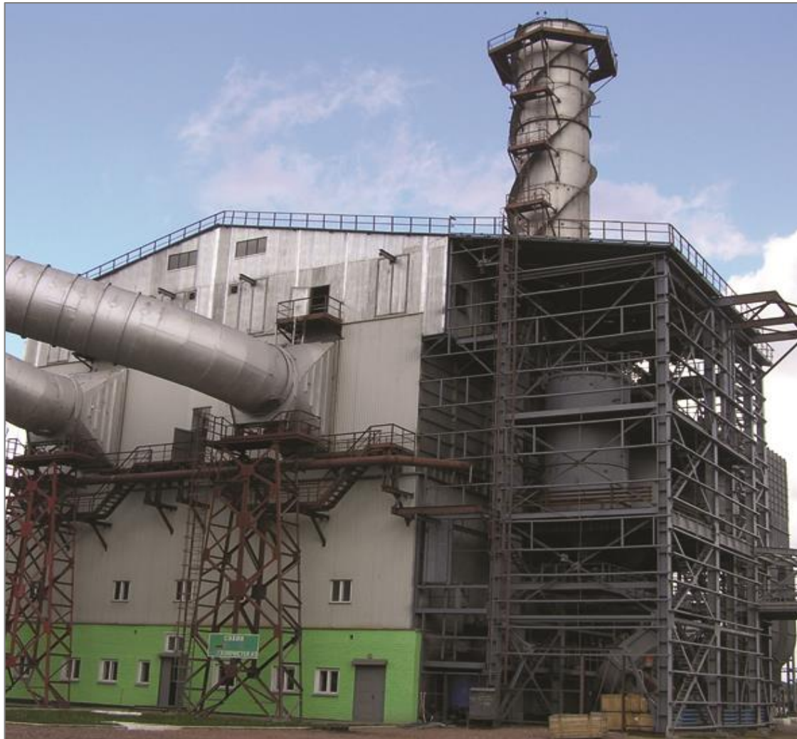
Bag filter for ferroalloy furnaces №5 and 6
